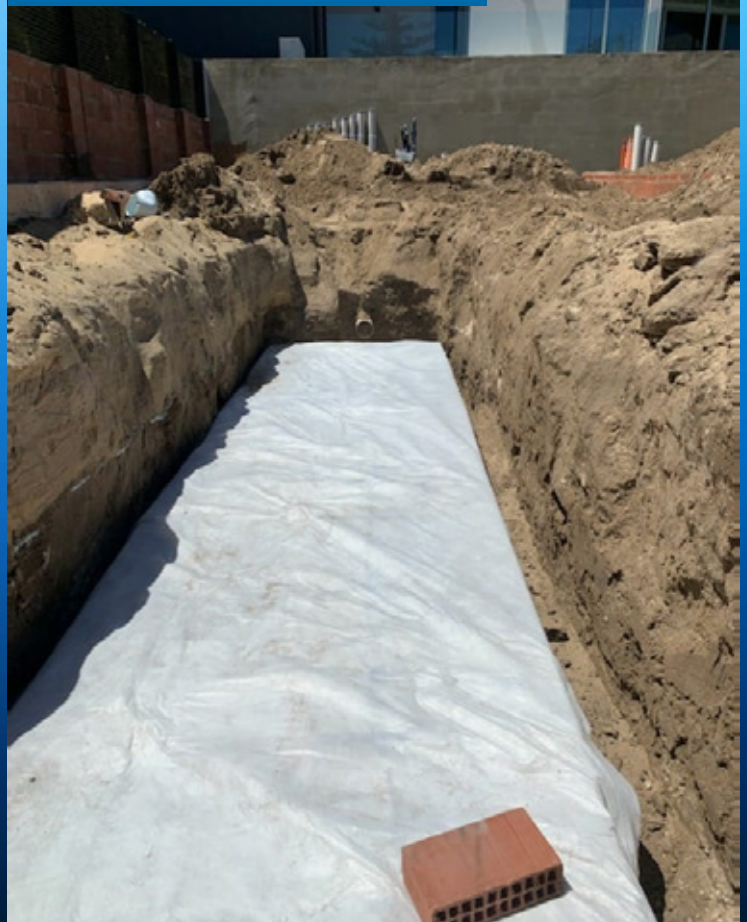
Tank Wrapped, Ready For Backfill
