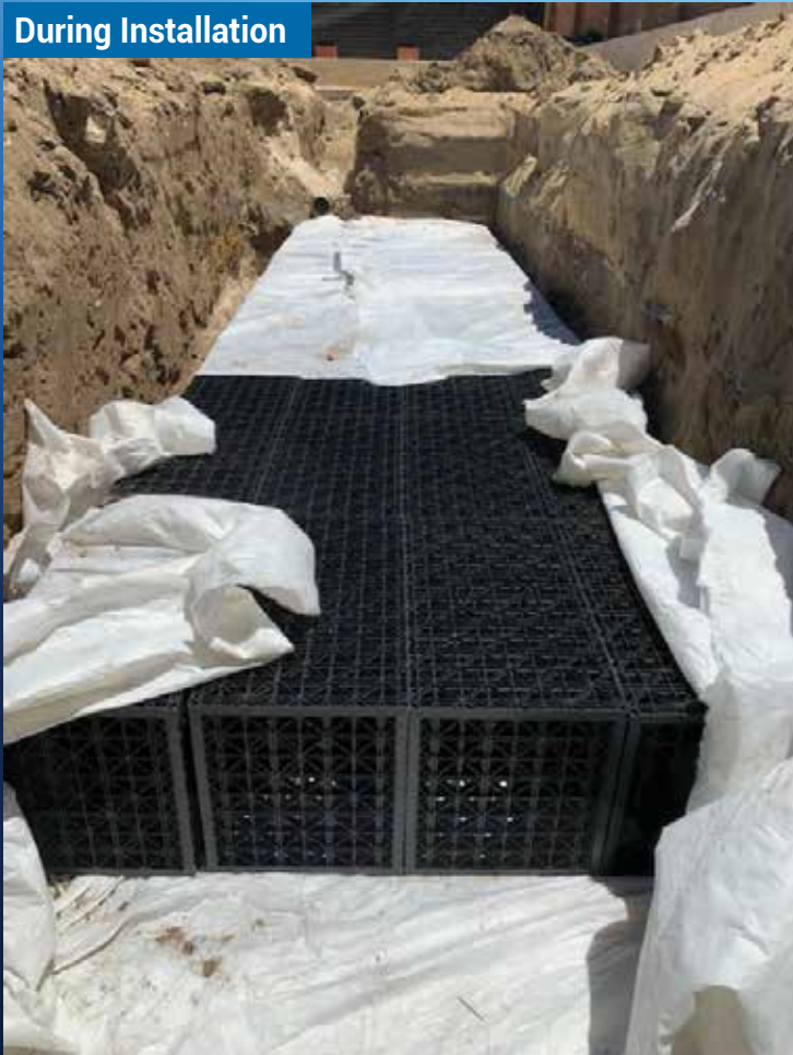
Tank Wrapped, Ready For Backfill
