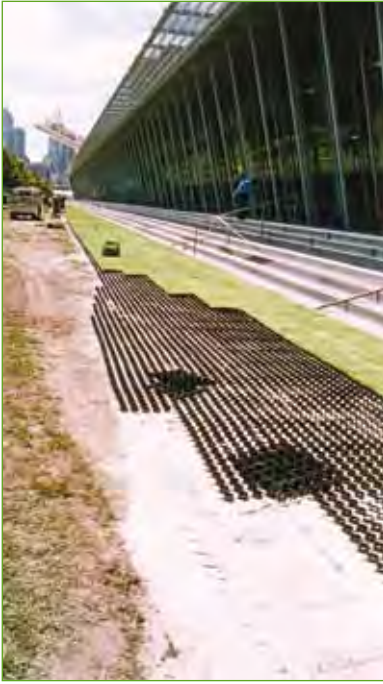
Melbourne Exhibition Centre during installation
