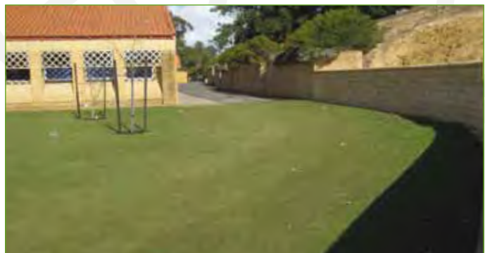
Service vehicle access, installed using Grassrings turf-reinforcement
